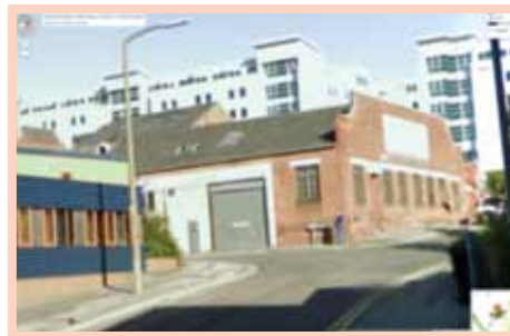
Before Works: Warehouse
