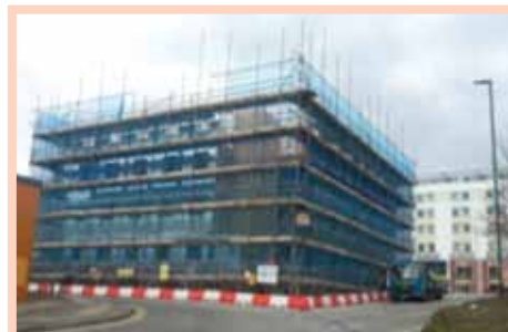
During Works: Conversion to Flats
